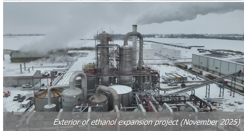
Exterior of ethanol expansion project (November 2025)
